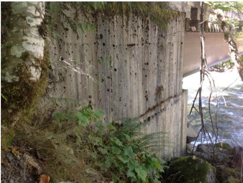
upstream left bank wing wall
