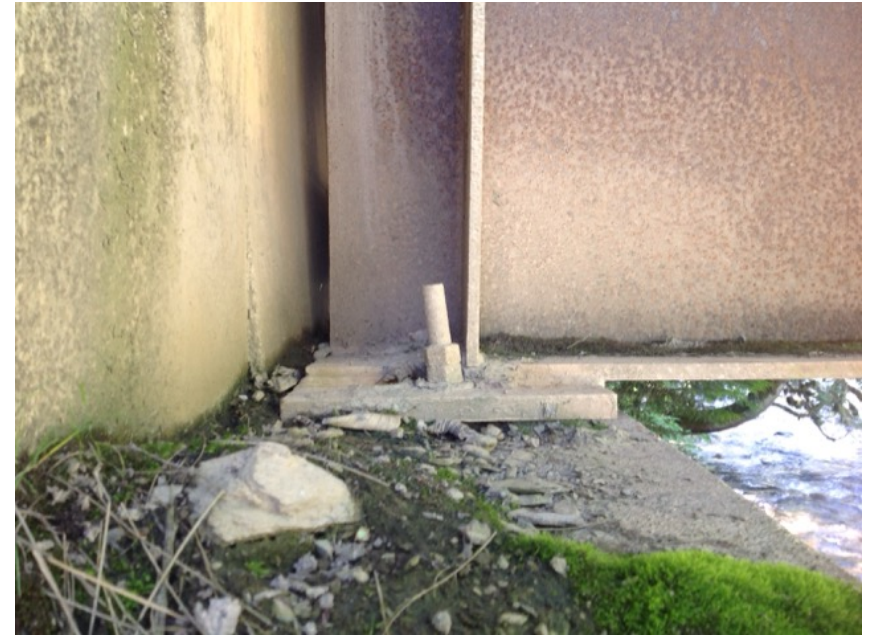
upstream left bank bearing
