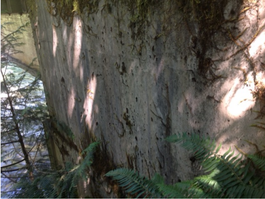
downstream left bank wing wall
