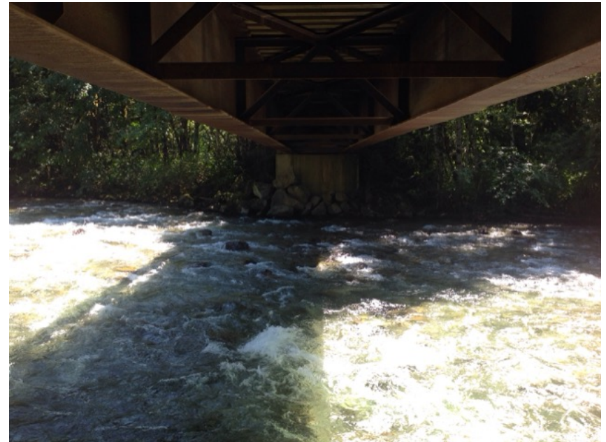
Left Bank Abutment when facing downstream
