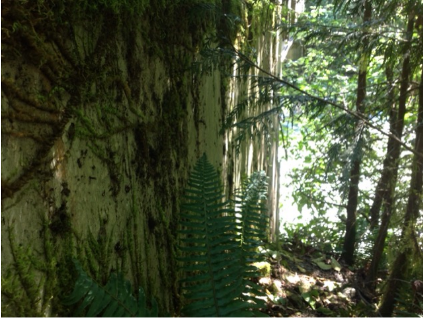
downstream right bank wing wall
