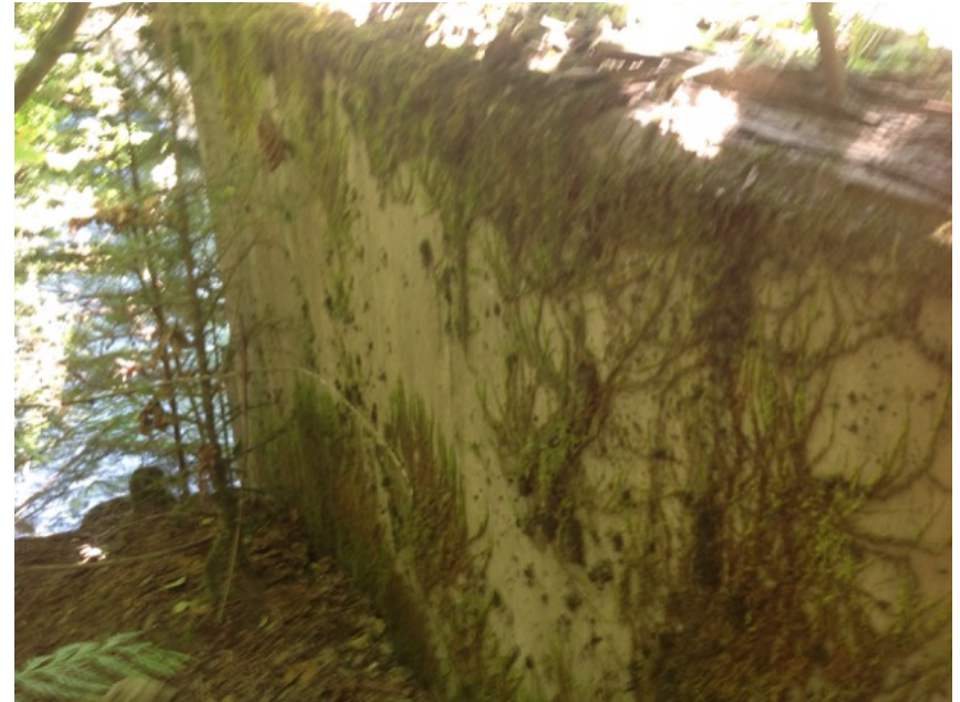
upstream right bank wing wall
